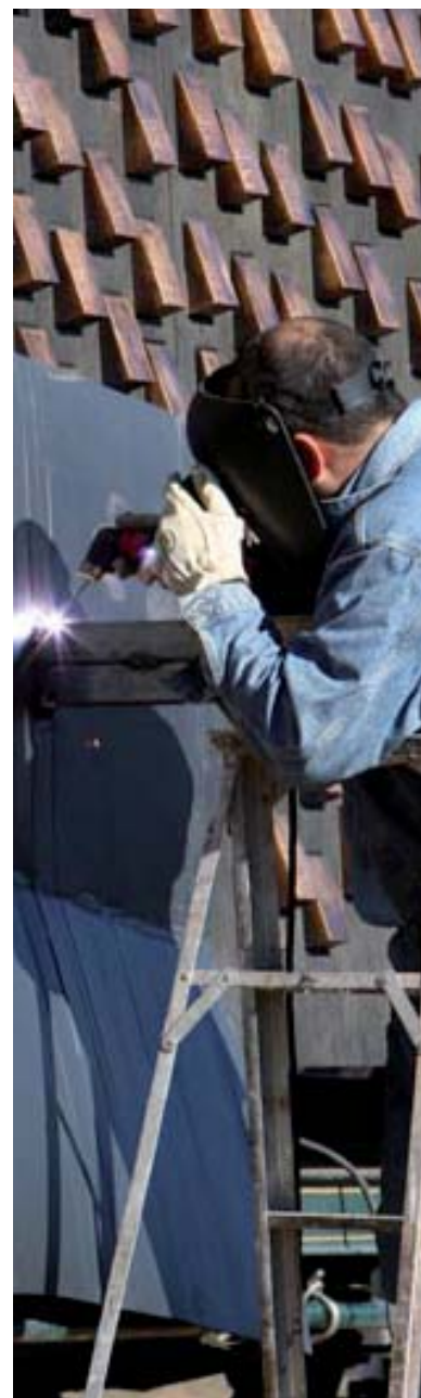
Construction of the memorial neared completion in August.
